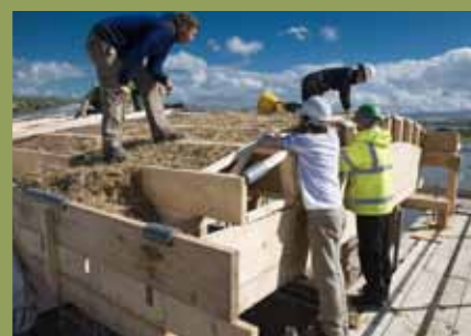
Filling The LookOut roof with straw
