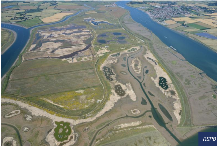
75. An aerial view of most of Wallasea Island, Essex, looking west, July 2019.
