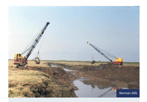
**79.** View looking west over the main tidal creek ('The Gut') as it is being filled to carry the new bank, RSPB Titchwell, Norfolk, 1975.
